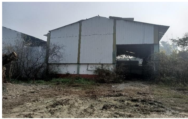
Figure 43 Rajau Paraspur SWM Plant
