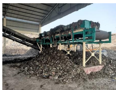
Figure 45 Treatment facility in Bakarganj SWM plant
